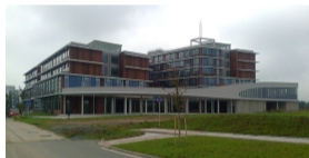
(b) FAV building
